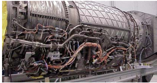
Figure II-25. Fire Suppression Duct Work Around a Military Aircraft Engine Nacelle.
